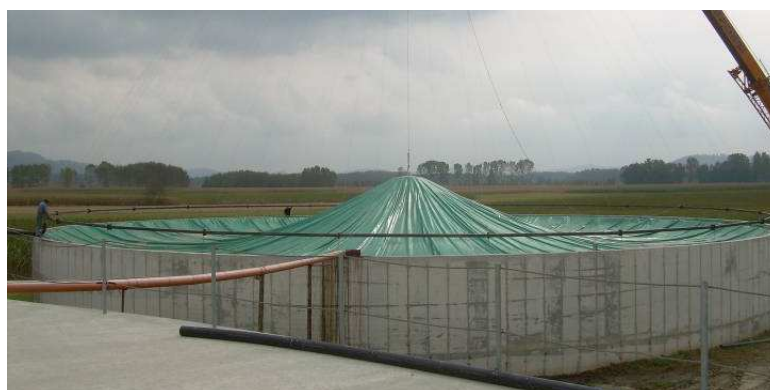
Fig. 6 – The floating cover system of the digestate storage tanks.
